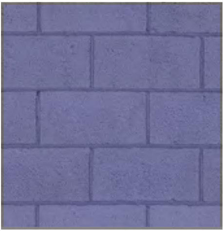
PAINTED CMU WALL
