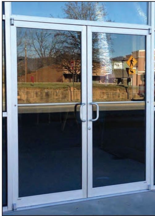
STOREFRONT SYSTEM BASIS OF DESIGN: OLDCASTLE STYLE: FG-3000 FINISH: PPG DURANAR XL UC51131XL SILVER
